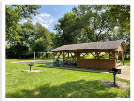
Existing Picnic Shelter
