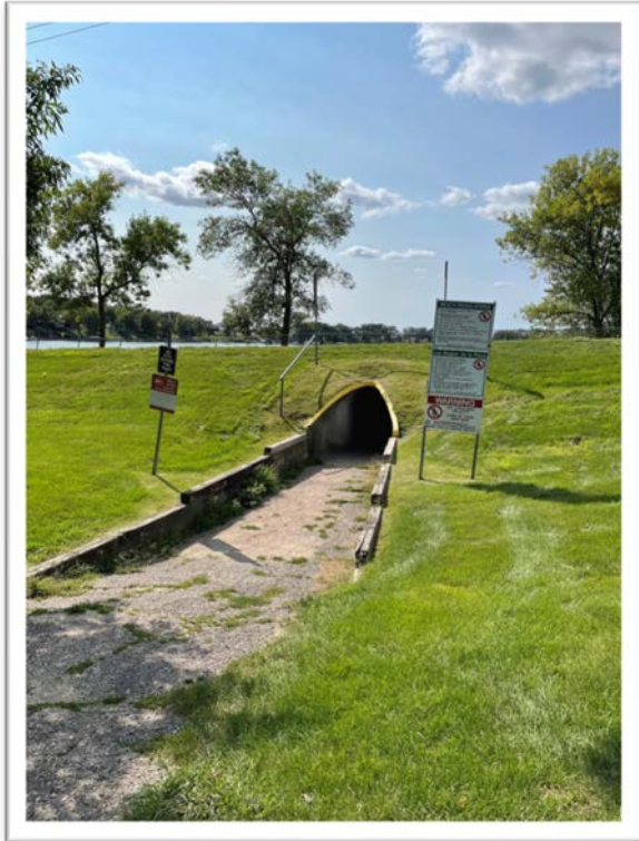
Existing Pedestrian Tunnel
